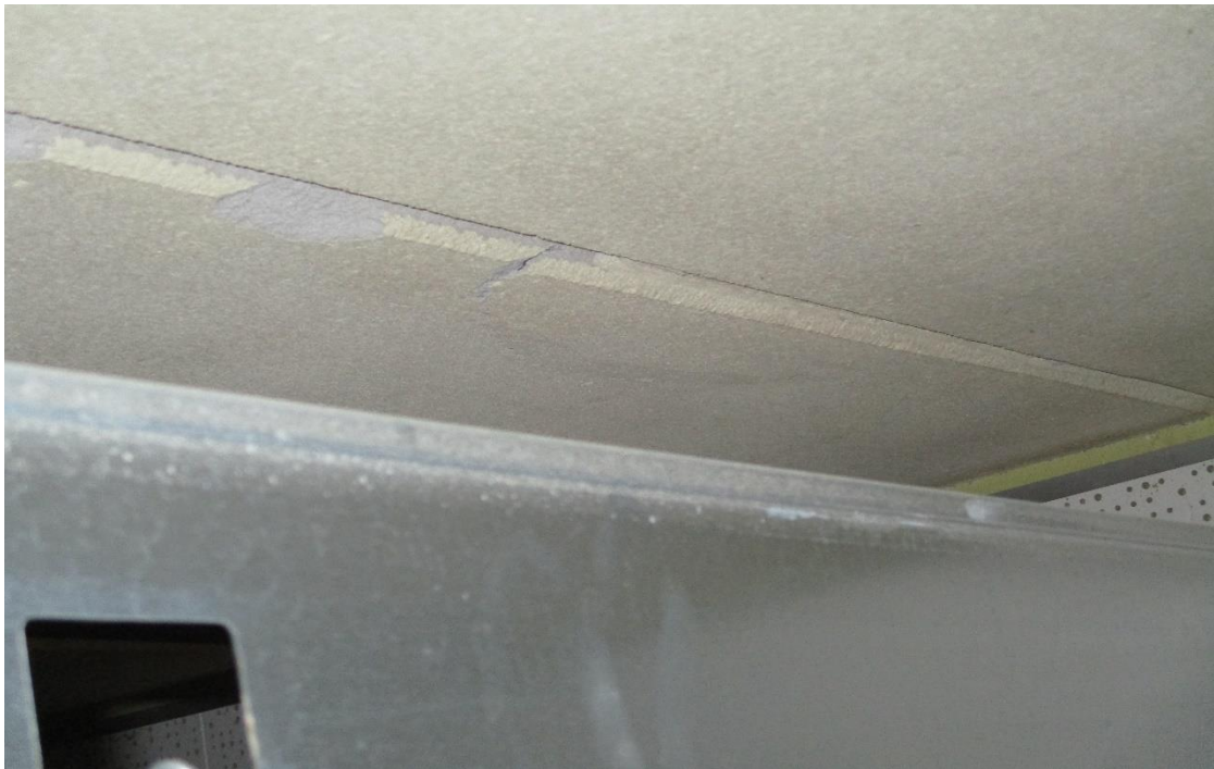
Delamination of Slabs
