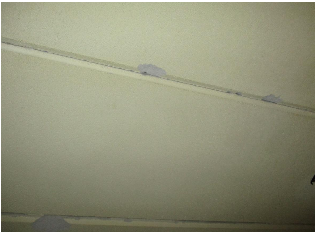
Spalled Edges
