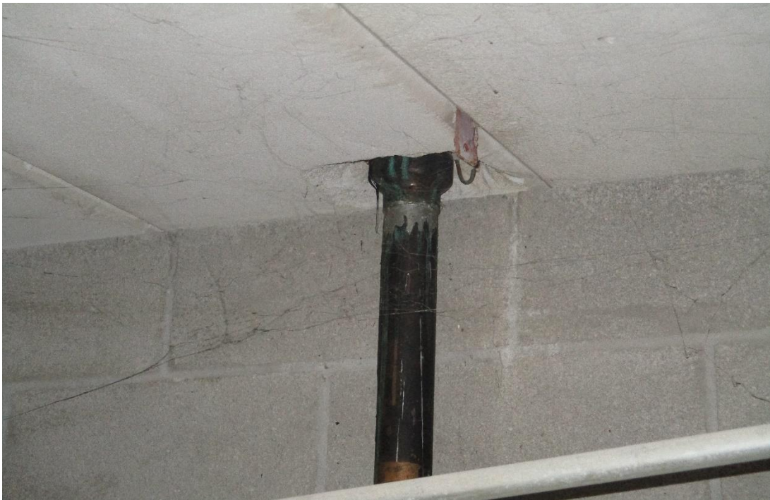
Improper Drain Penetration
