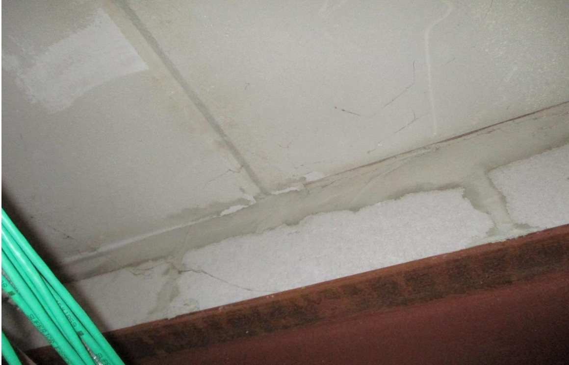
Previous Repair with Grouting
