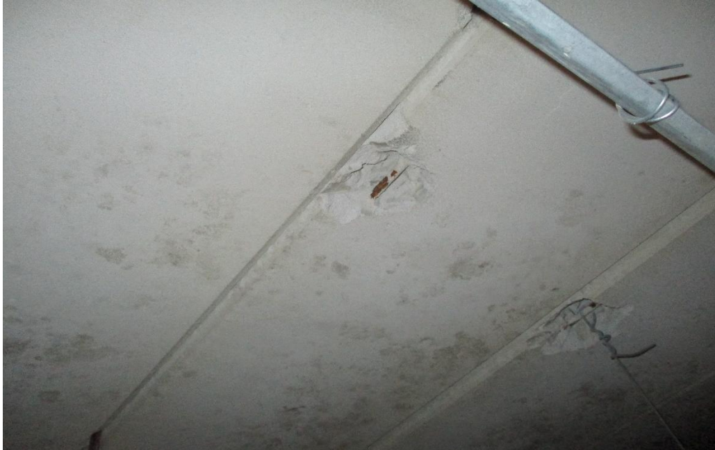
Chipping and Gouging
