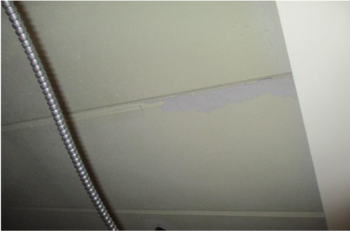
Delamination of Slabs
