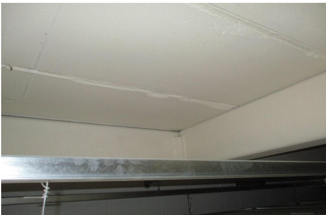
Delamination at Edges
