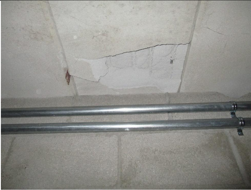
View of major area of spalling RAAC panels
