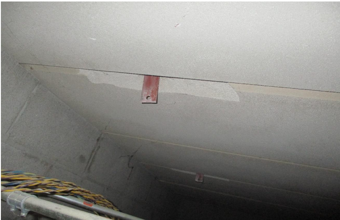
Large Gouge around Hanger
