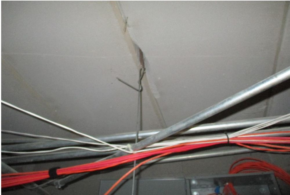
Improper Hanger
