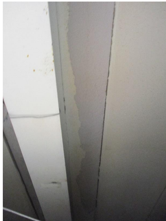
Large Surface Delamination
