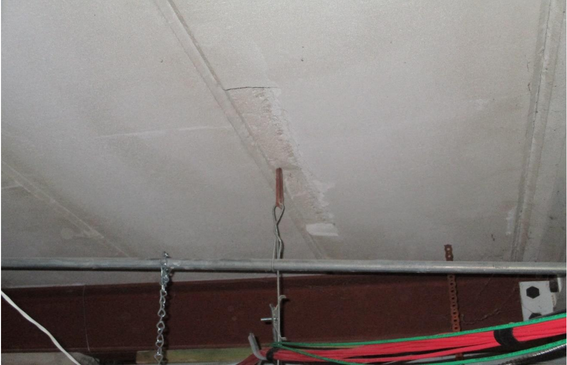
Delamination of Slab
