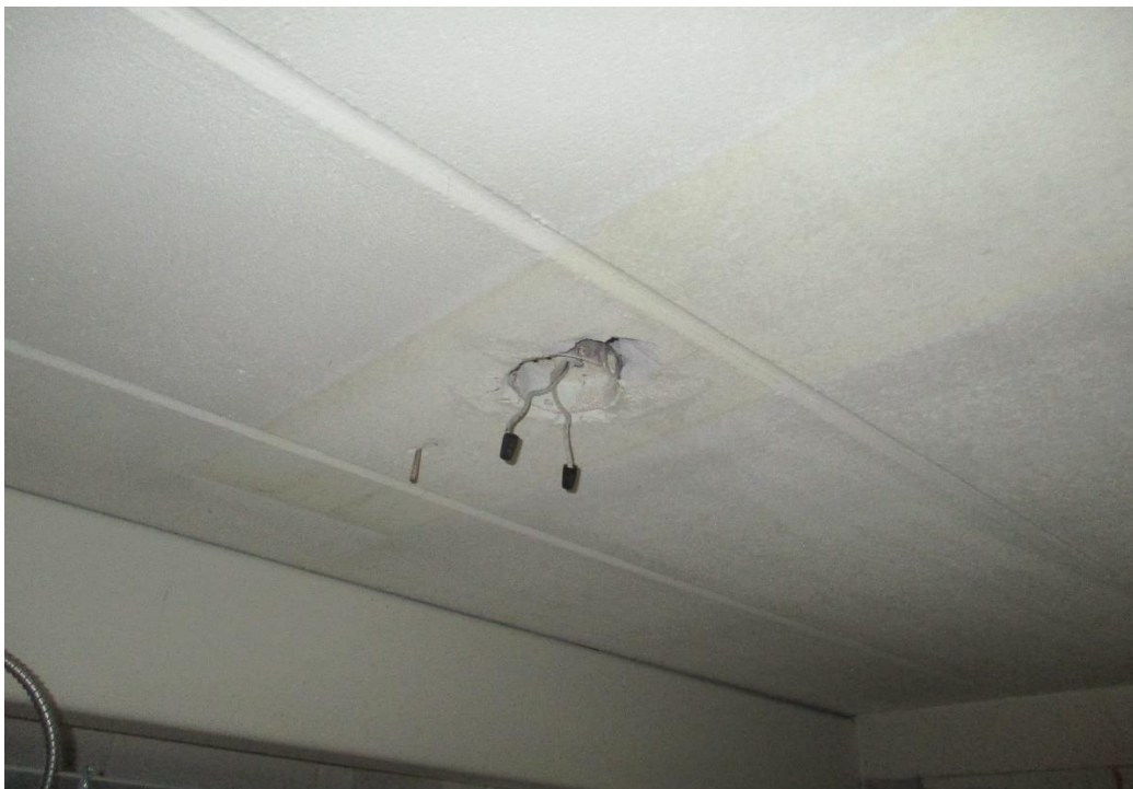
Improper Fixture Installation
