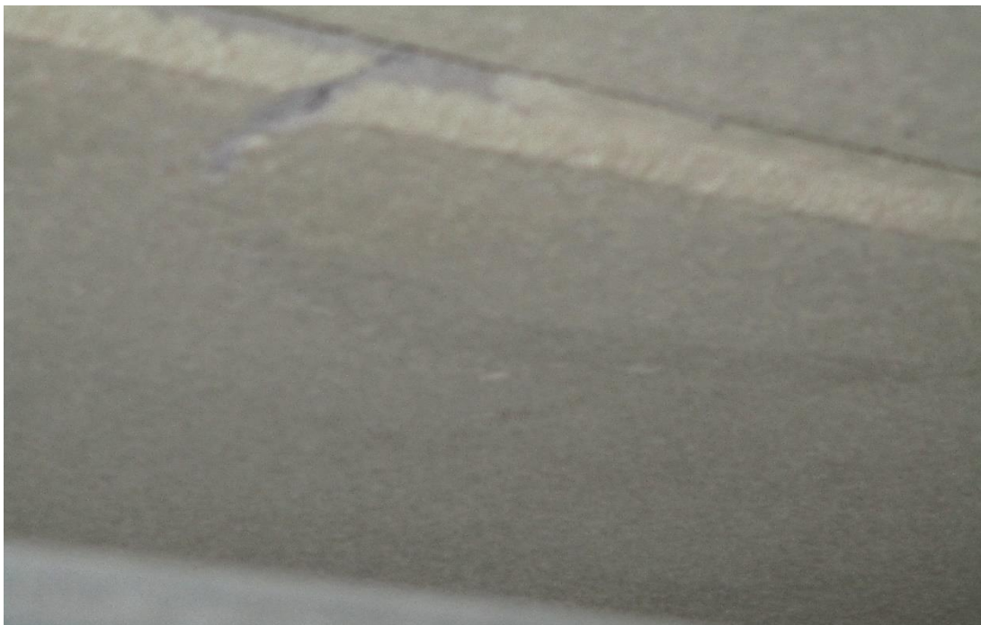
Delamination of Slabs
