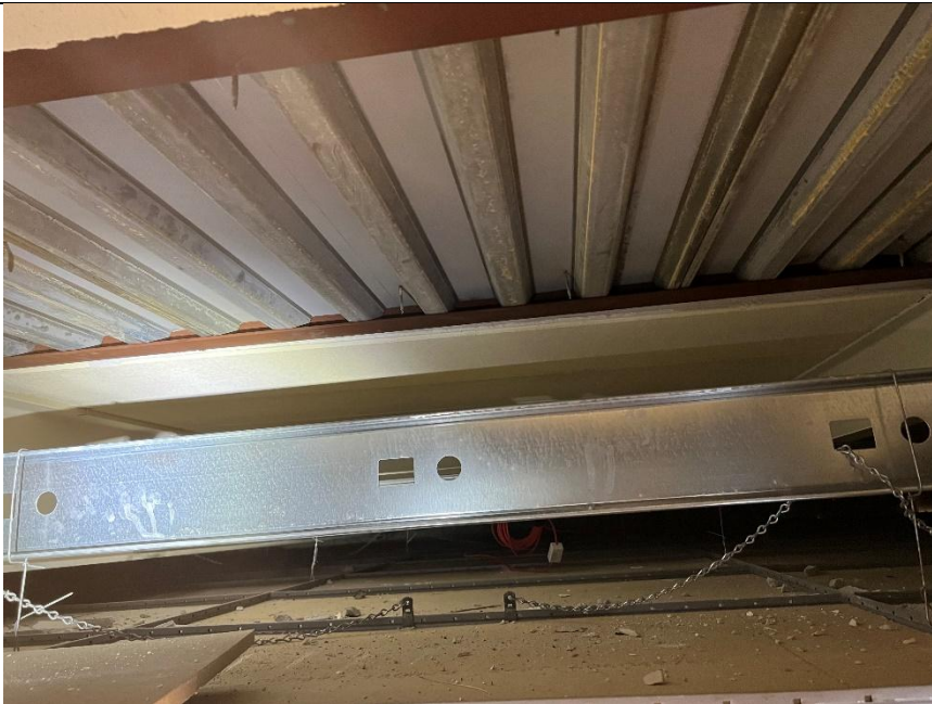
View of former RAAC replacement in Classroom
