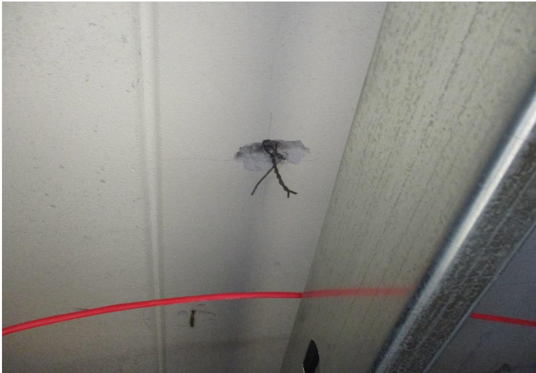
Improper Hanger
