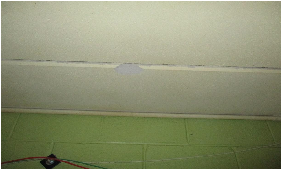
Spalled Edges
