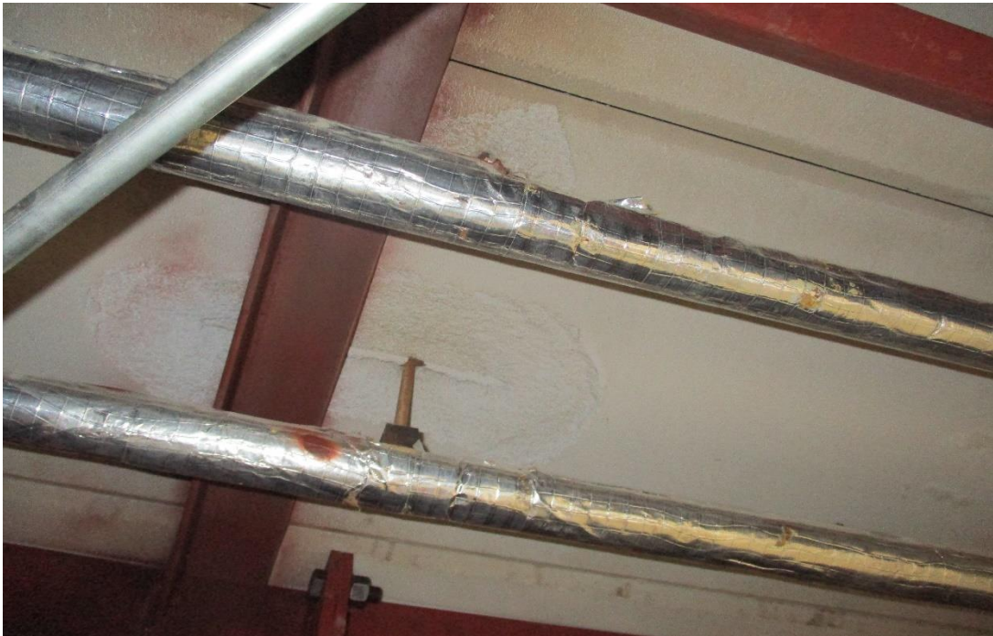
Delamination of Slab
