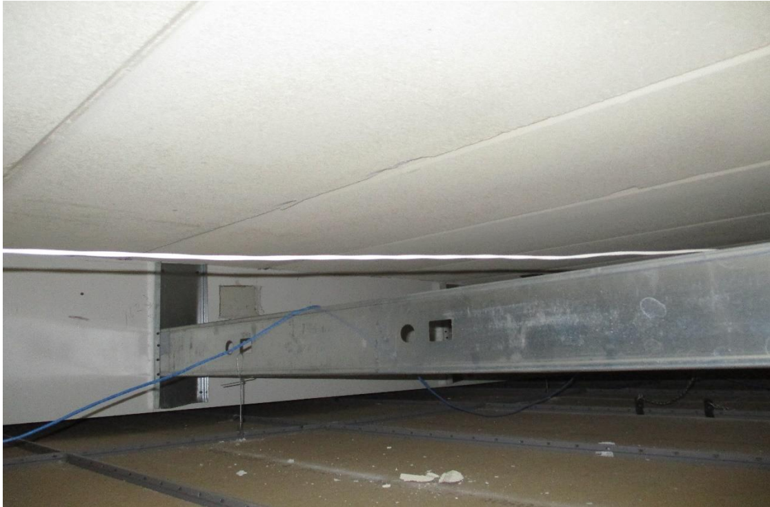
Delamination of Slabs
