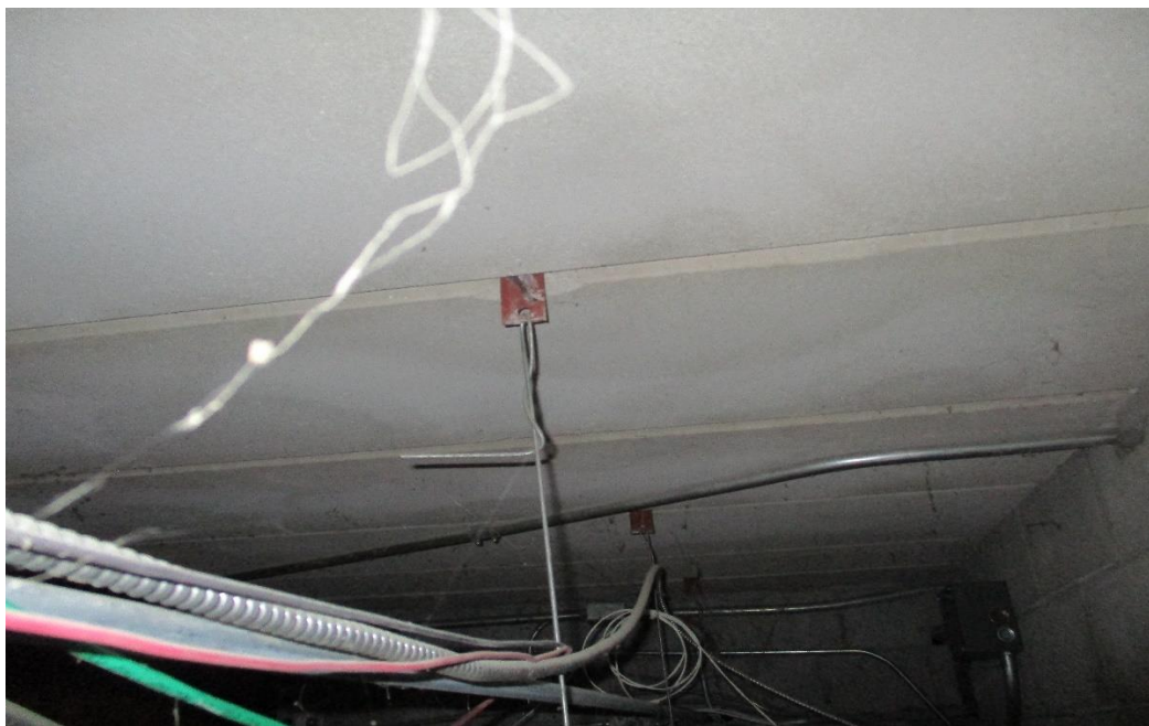
Improper Hangers/Chipping
