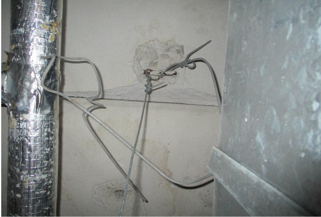
Improper Hanger
