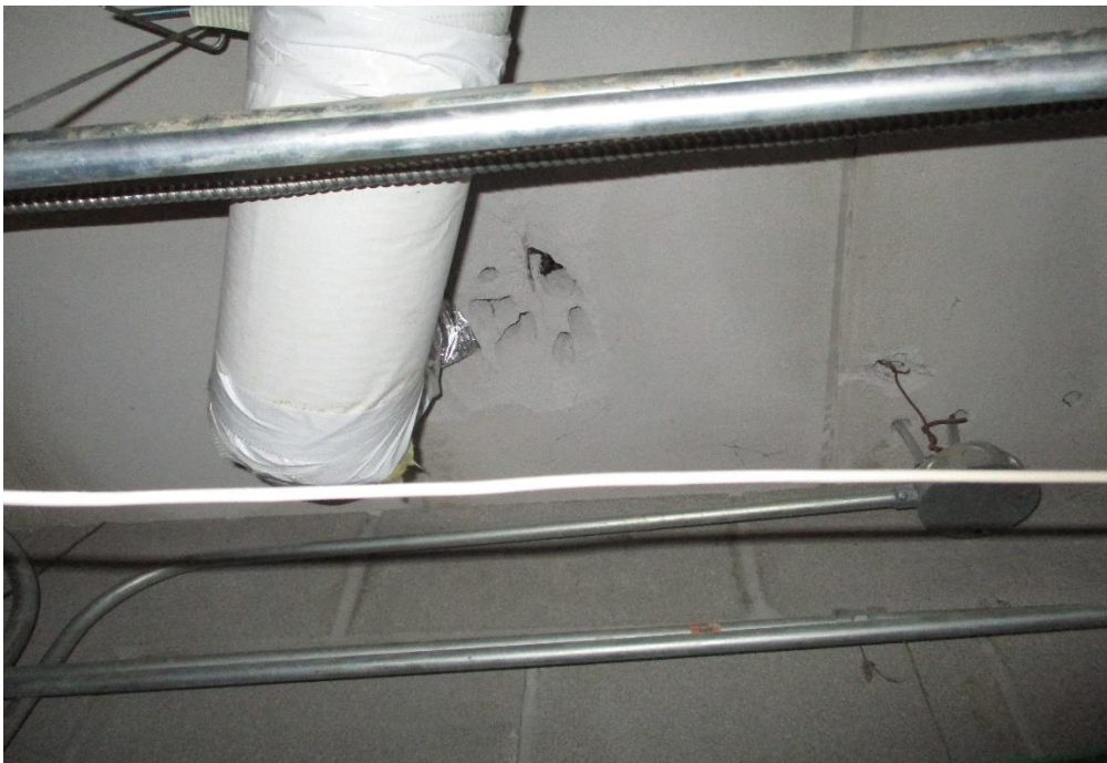
Chipping and Gouging
