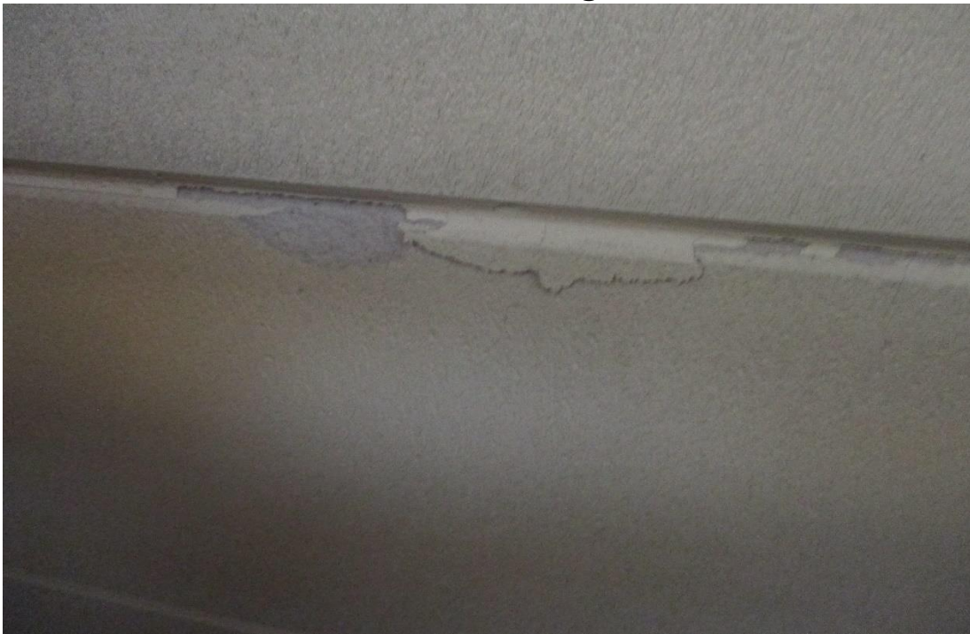
Delamination at Edges
