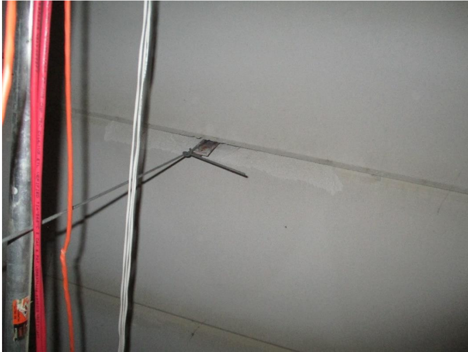
Improper Hanger
