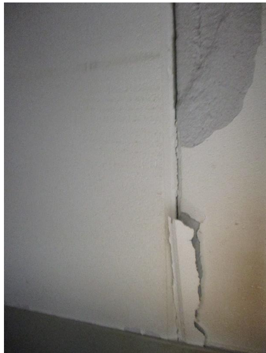
Severe Delamination and Cracking
