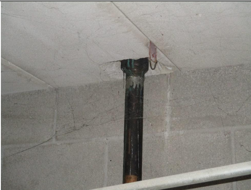
View of improper opening and hanger in RAAC panels
