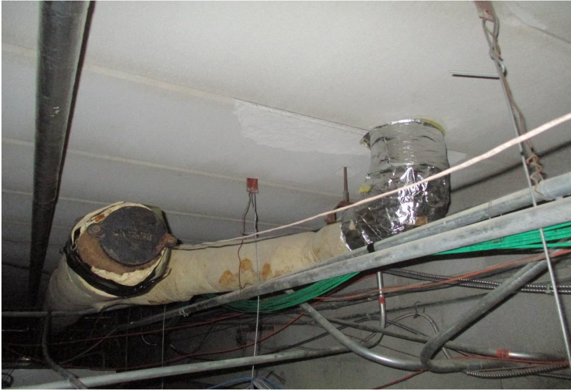
Large Surface Delamination
