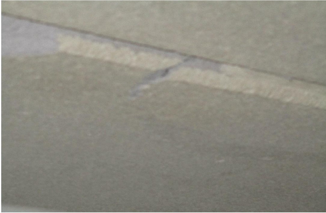
Delamination of Slabs
