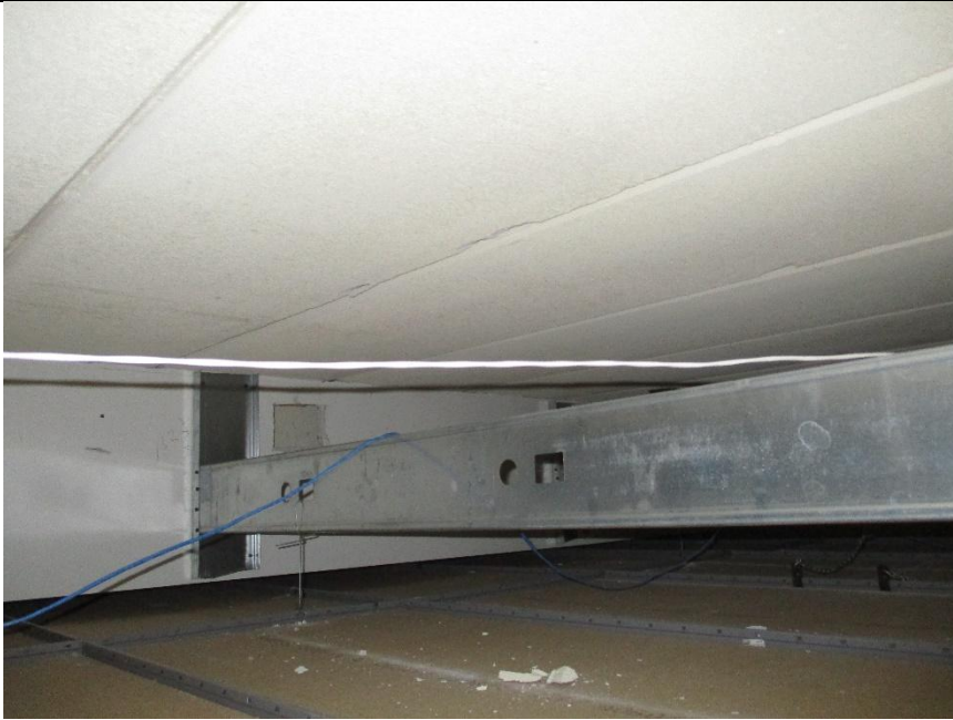
View of secondary framing below RAAC panels to support ceiling
