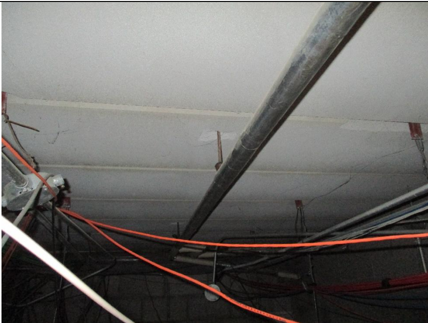
View of improper hanger in RAAC panels
