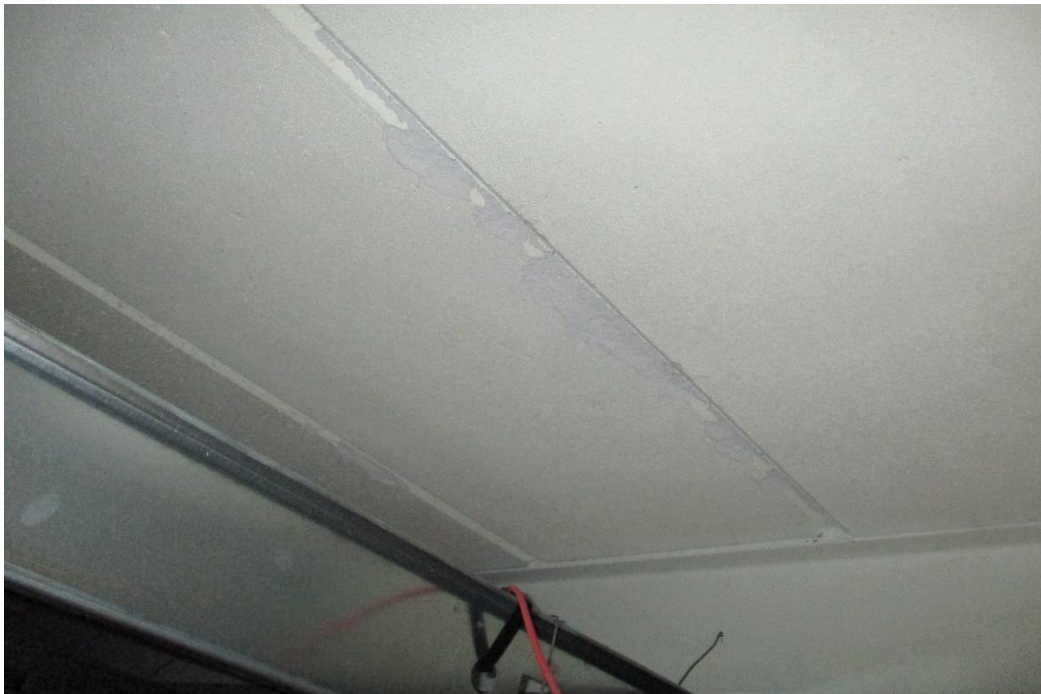
Delamination/Missing Grout
