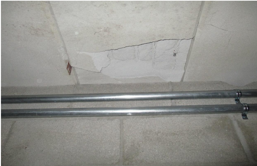
Large Surface Delamination
