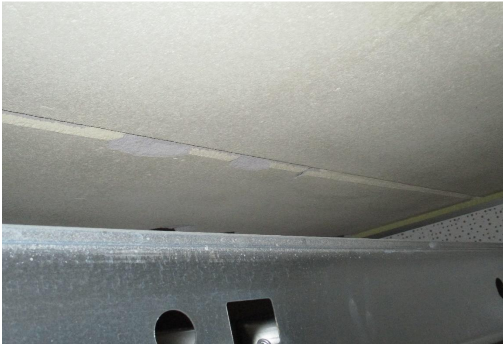
Delamination of Slabs
