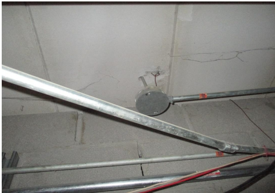
Improper Service Penetration
