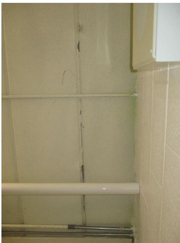
Delamination/Missing Grout
