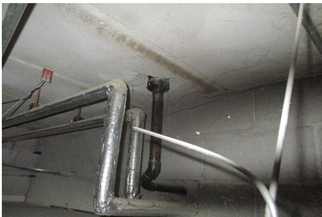
Roof Drain Penetration Not Framed
