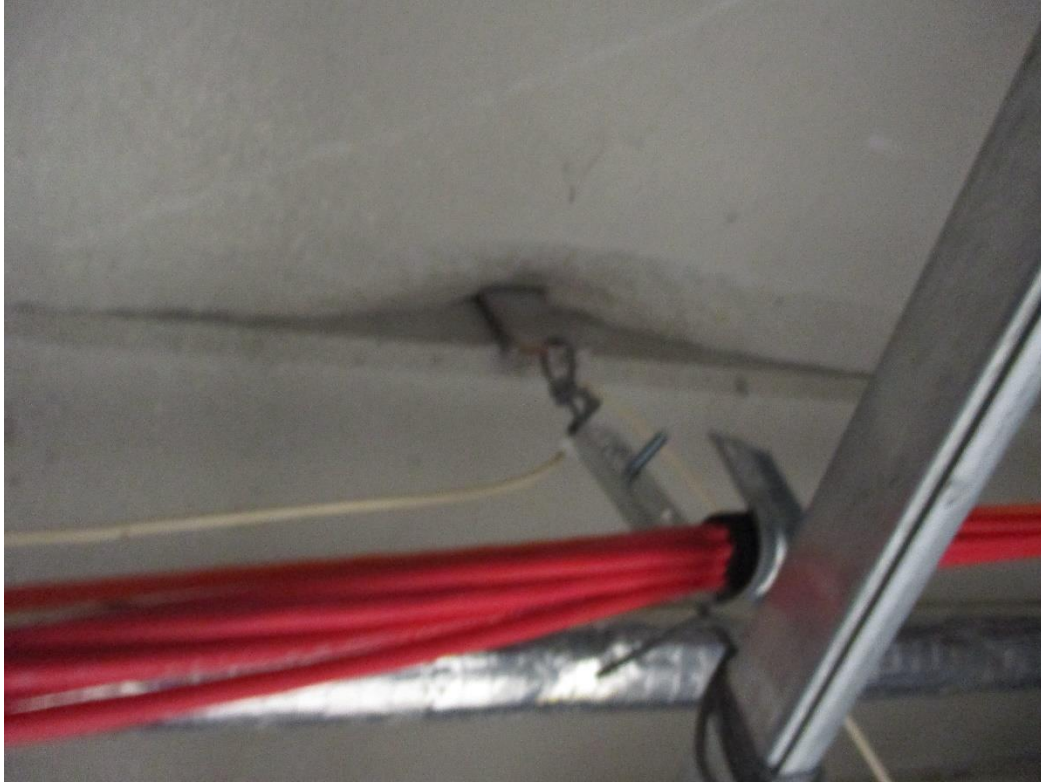
Improper Hangers/Chipping
