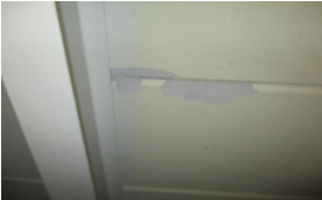
Delamination of Slabs
