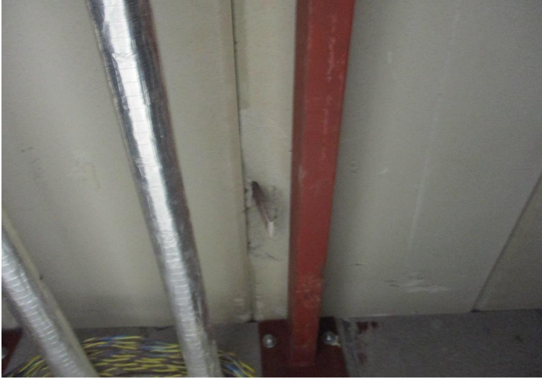
Improper Hanger
