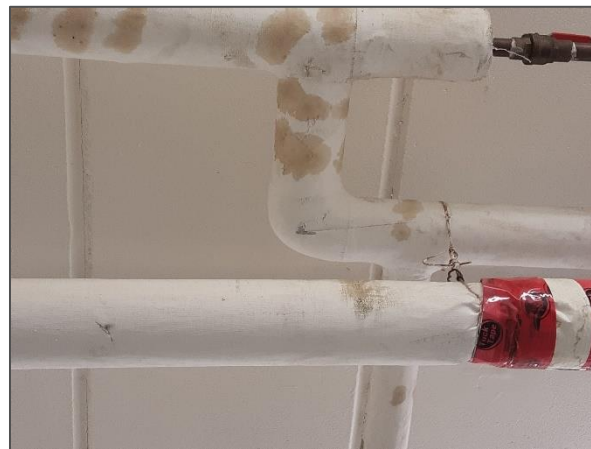
Asbestos-containing parging cement pipe insulation.
