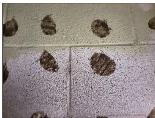
Non-asbestos brown wall mastic.
