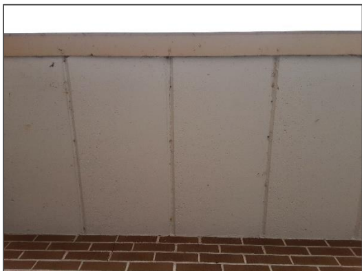
Asbestos-containing Siporex panels.
