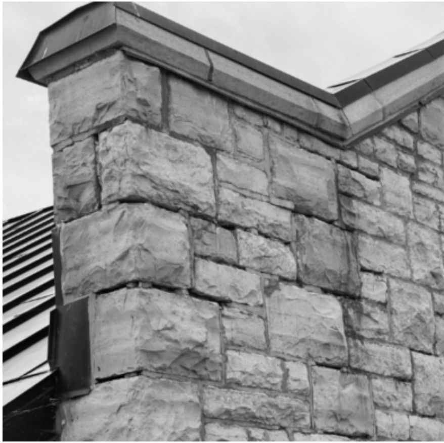
2 FORT LASALLE ZONE 4 NORTH ELEVATION - REBUILD, REINFORCE GABLE END PARAPETS SCALE: 1:1
