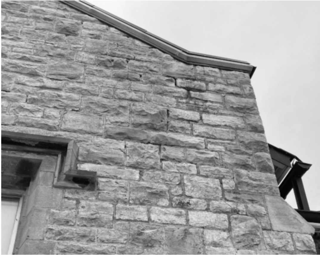
6 FORT LASALLE ZONE 2 S-E PROJECTING BAY - REBUILD WALL - REPLACE 5 STONES AND REPAIR METHOD 'E' SCALE: 1:1
