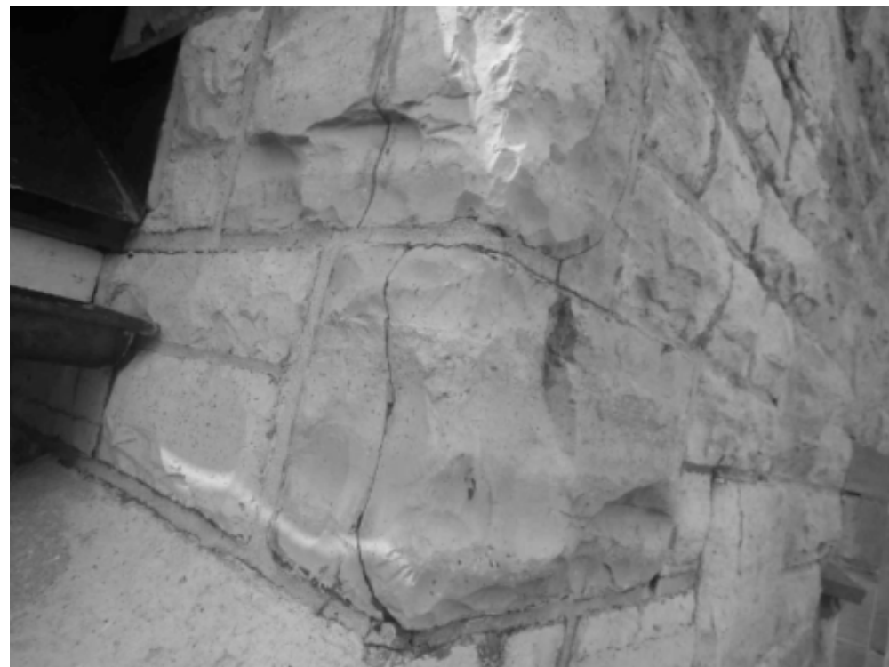
BULLNOSED CORNER STONES WITH DEFINED VERTICAL LEDGE. NO MARGIN OR BUSHHAMMER
