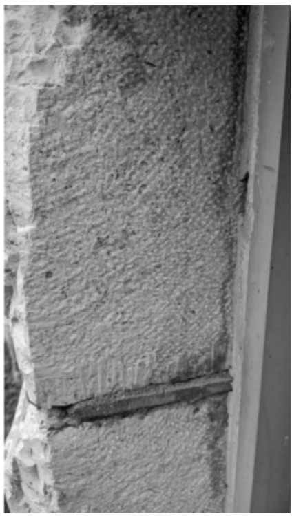
BUSHHAMMER AND MARGIN AT WINDOW JAMBES
