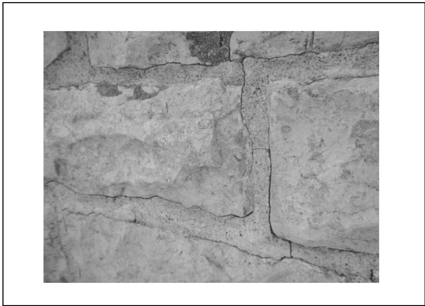
1 206 FORT LASALLE METHOD A1 - UP TO 49mm REMOVAL OF SOUND MORTAR SCALE: 1:1
