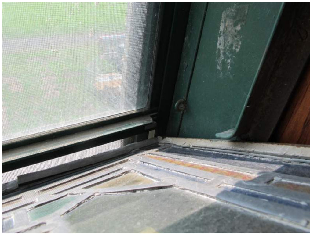
8 304 NTS TYPICAL CONDITIONS AT HOPPER VENT AND EXISTING STORM WINDOW
