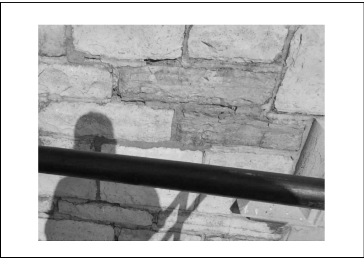
1 205 YEO HALL METHOD 'A1' UP TO 49mm REMOVAL TO SOUND MORTAR SCALE: 1:1
