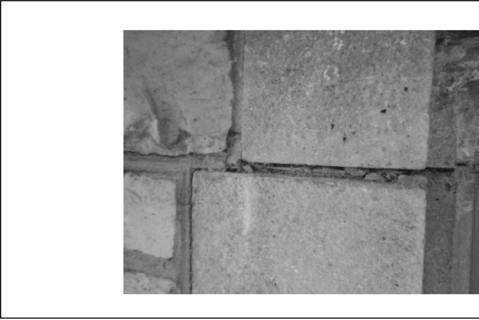
1 205 YEO HALL METHOD 'A1' UP TO 49mm REMOVAL TO SOUND MORTAR SCALE: 1:1
