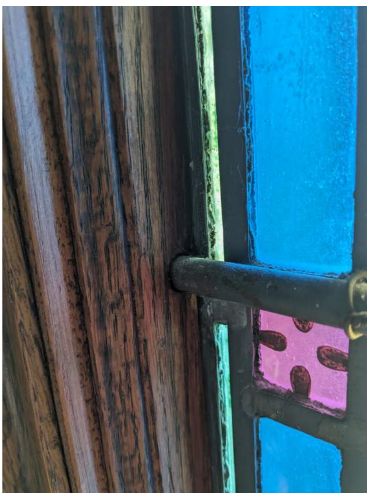
10 304 NTS TYPICAL SADDLE BAR MOUNTING IN FRAME
